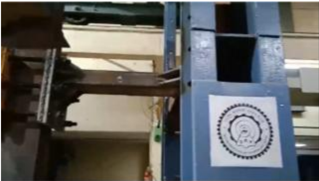
Bridge between Damper and Moment Resisting Frame
